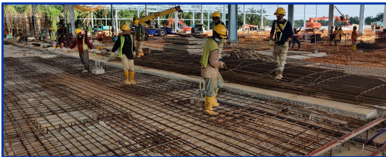
Figure 2.9.1: Laying of SSM Bar Mat for slab
